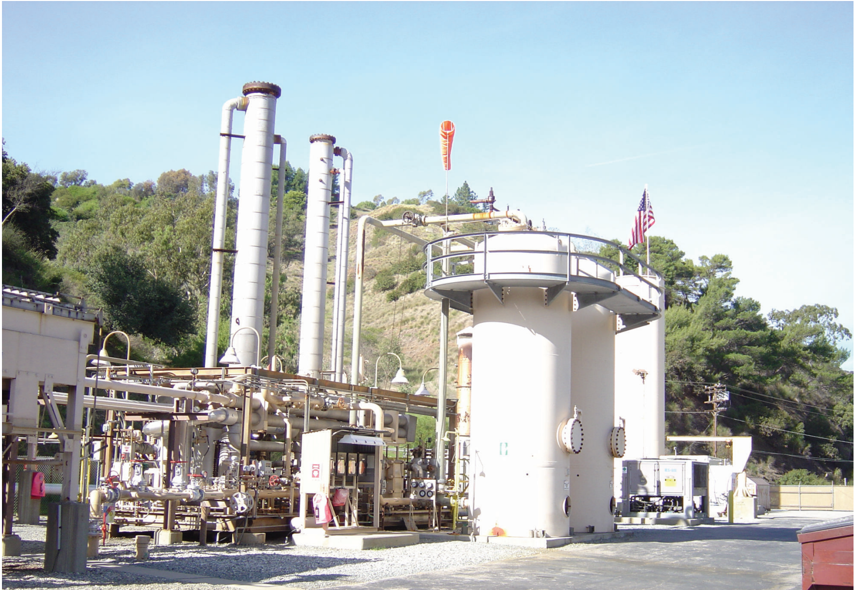
FIGURE 5 - Typical LFG Medium BTU Gas Processing System
