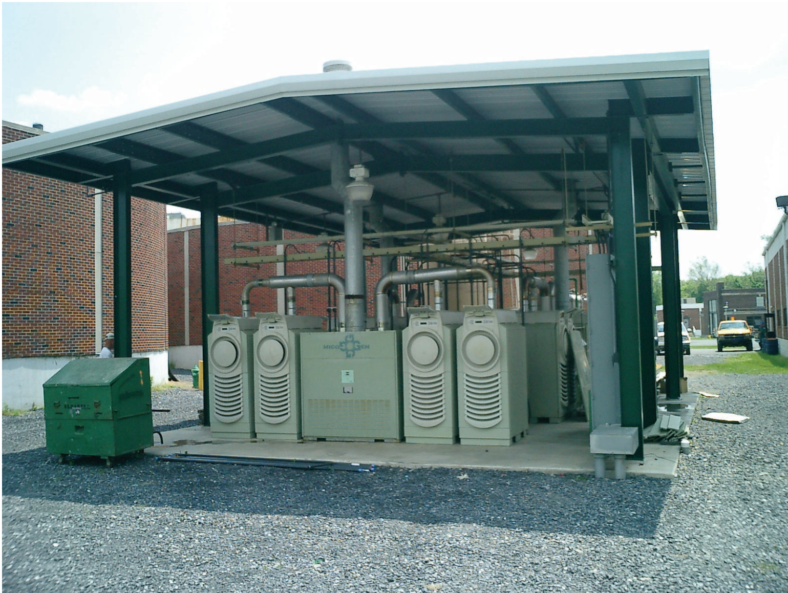
FIGURE 9 - LFG Electricity Generating Facility Using 12 30-KW Capstone Microturbines
