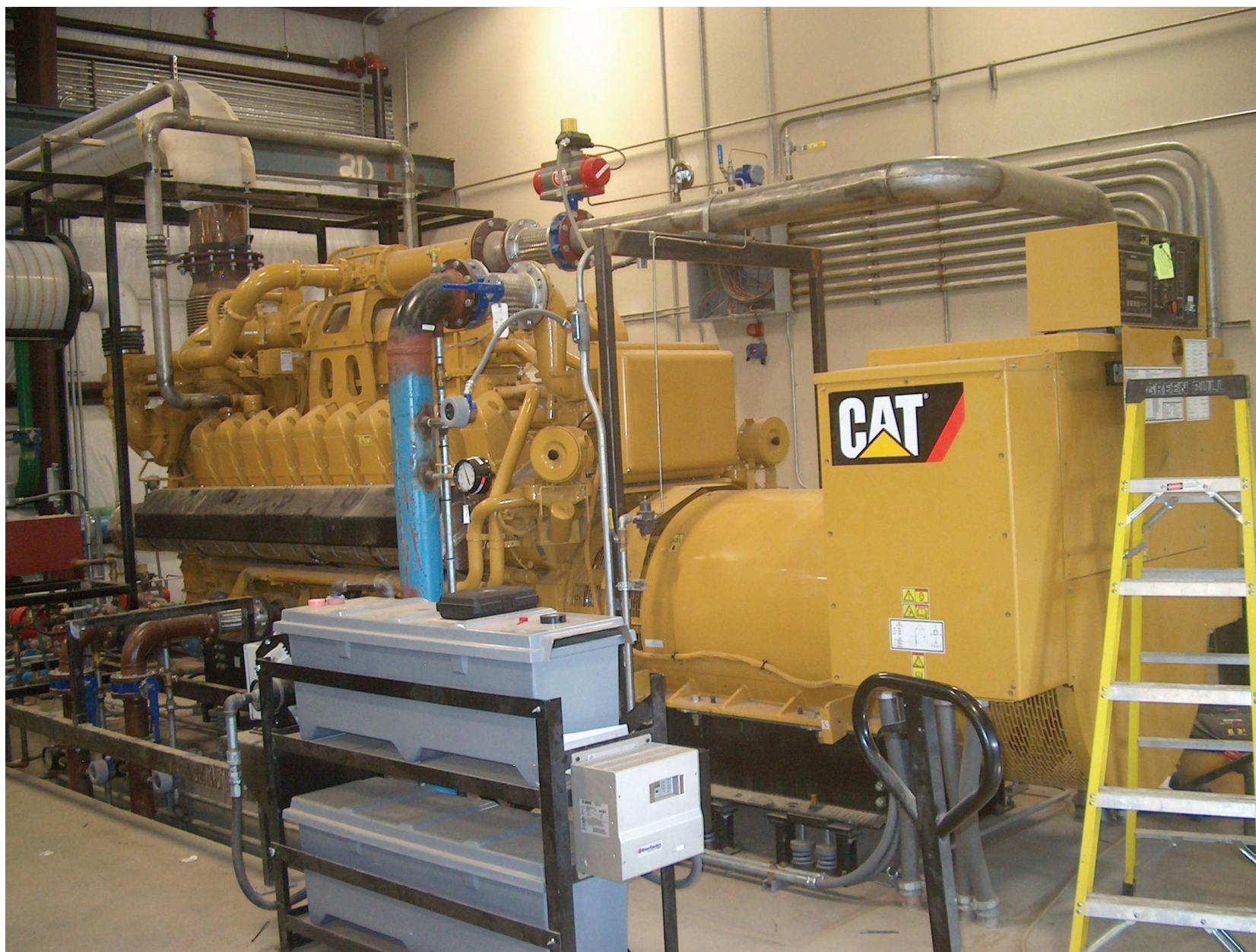
FIGURE 7 - Caterpillar LFG Engine-Generator Set
