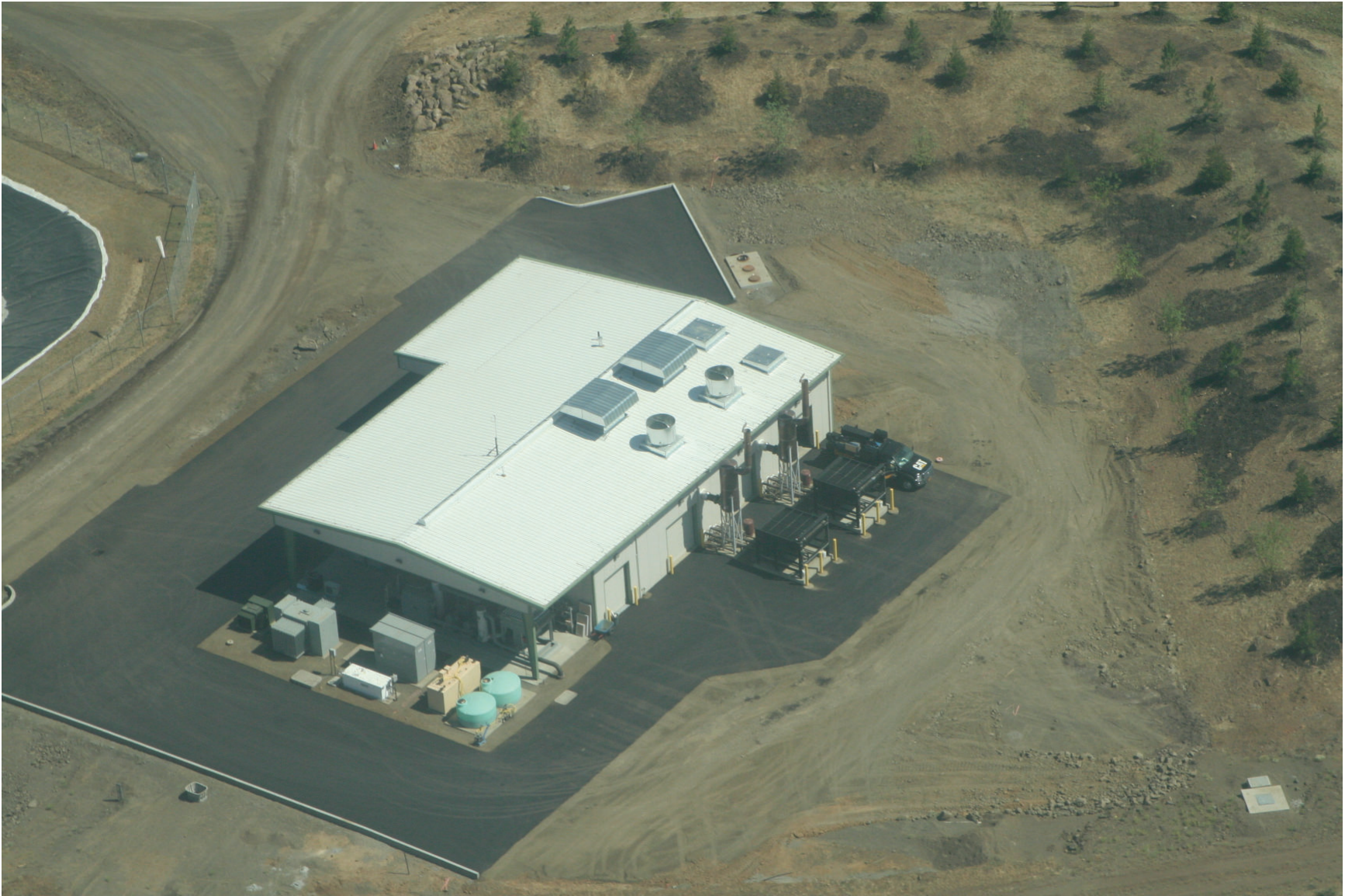
FIGURE 8 - Typical LFG Electricity Generating Facility Using Internal Combustion Engine-Generator Sets
